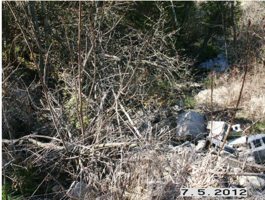
Photo 9 – Culverts and other debris impact the connectivity of the south tributary just downstream (west) of the site
